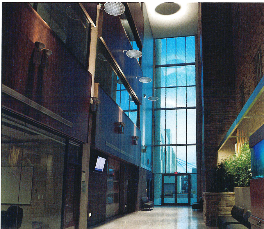
A SERIES OF DISCS REFLECT DAYLIGHT TO THE LOWEST LEVEL OF THE ATRIUM. IN THE EVENING THE DISCS BOUNCE LIGHT FROM HIGH EFFICIENCY LED SPOT LIGHTS BACK DOWN TO THE FLOOR [4].
